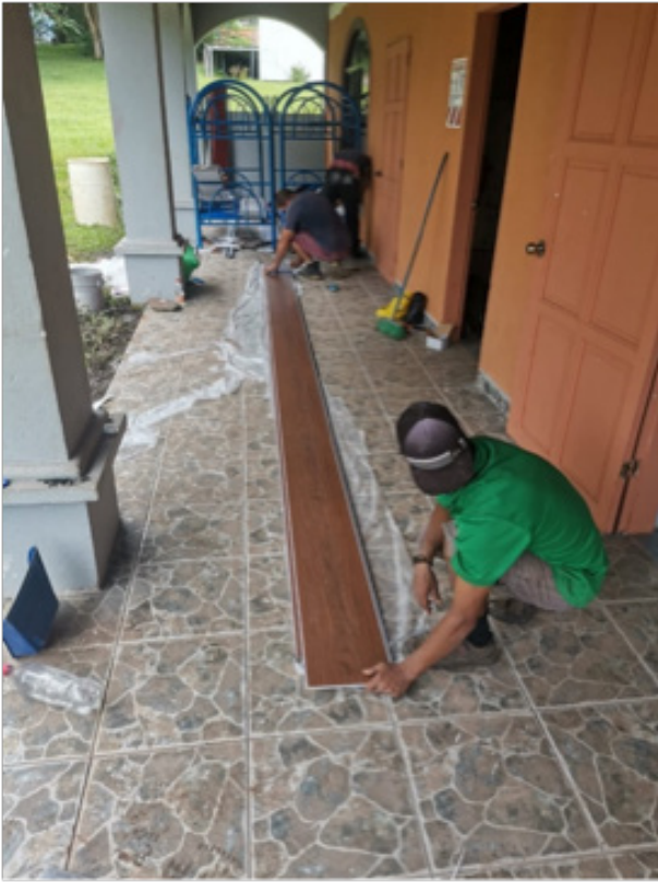
Many renovations and general repair took place during this past year.
