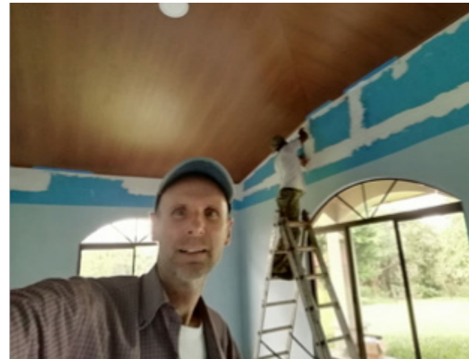
Ceiling replacement in the Boys' Dorm
